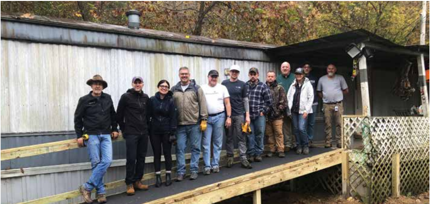
As part of the Healthy Homes project, a team from AdventHealth constructs a ramp to improve a resident’s access into their home.
