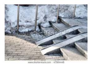
$<sup>^{1}1:12</sup>$  means for every 12 inches along the base of the ramp, the height increases one inch.
